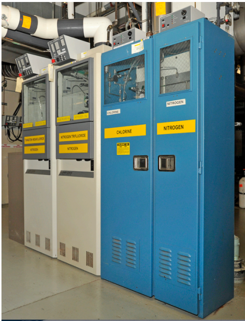
Toxic Gas Cylinders in Vented Toxic Gas Cabinets
