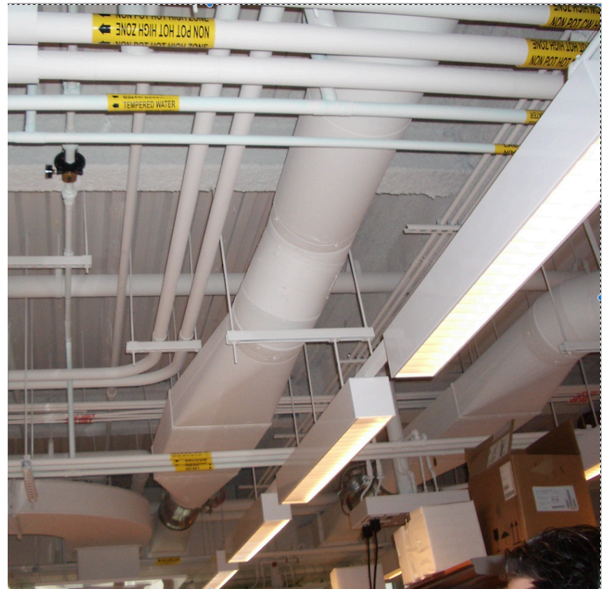
Automated Water Sprinkler System on Ceiling
