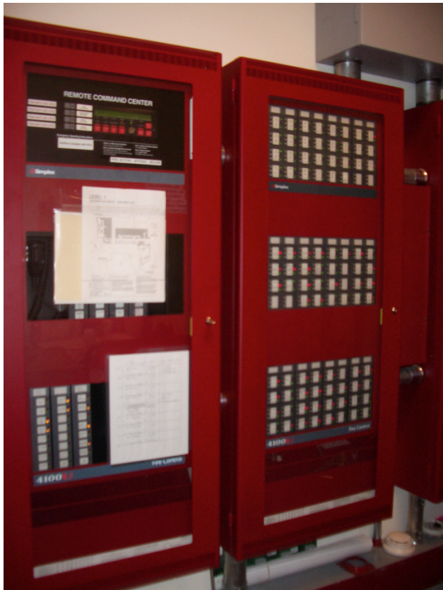
Fire Detection Control Panel in a Fire Department Control Center
